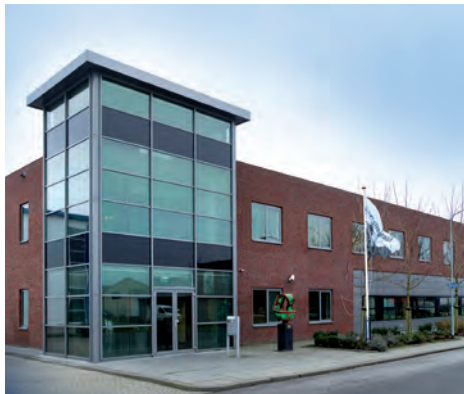
/ Centre for successful recycling technology: in Appingedam, a company consciously lives sustainability
